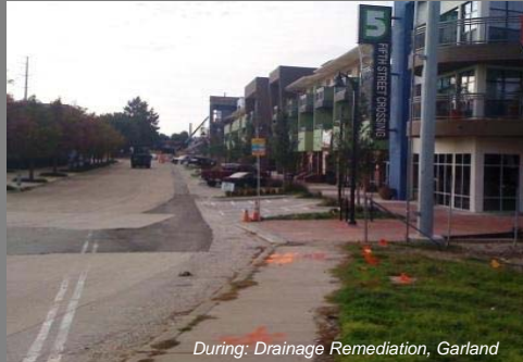
During: Drainage Remediation, Garland
