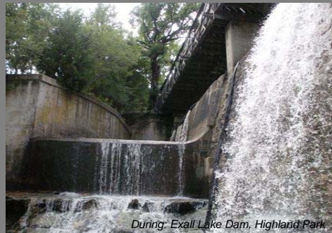
During: Exall Lake Dam, Highland Park
